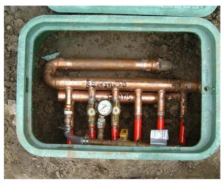
the concrete pour. Air pressure will vary due to outdoor air temperature so don't be alarmed if pressure in tubing has decreased the morning after installation. There should however still be air in tubing. If you feel you have a leak, check the manifold and test connections first.
