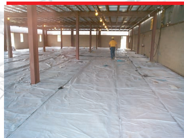
Insul-Tarp® as shown here, has been rolled out and installed with radiant tubing clipped to wire mesh.
